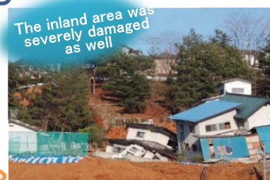
Status of housing damage (Fushigami, Fukushima City)
