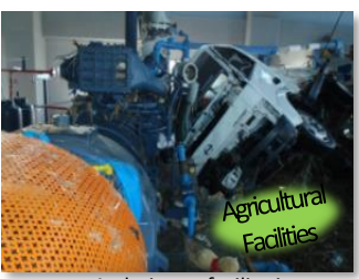
A drainage facility in Soma city Agricultural Facilities
