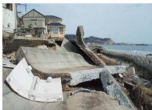
Iwaki City: Levee
