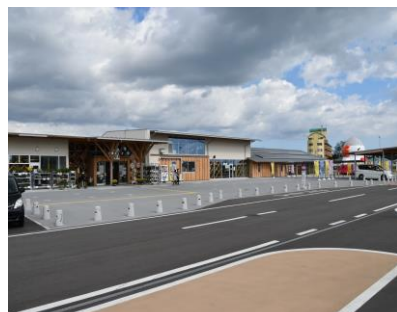
Namie Town: Roadside-Station "Namie"
