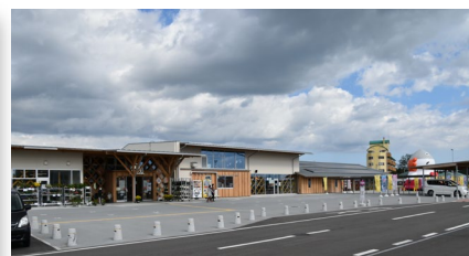
Namie Town: Roadside-Station "Namie"
