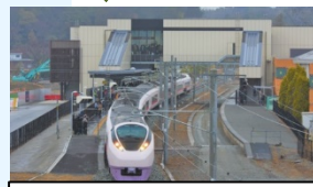
JR Joban Line Full operation of the line resumed on 14 Mar. 2020
