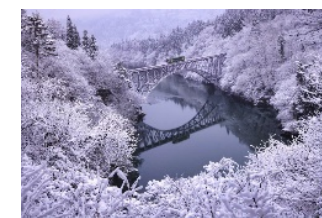
Tadami Line railway facilities
