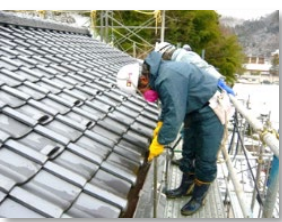
Decontamination of homes
