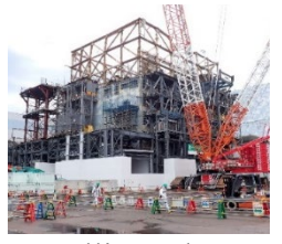
Installing a large cover for Unit 1
