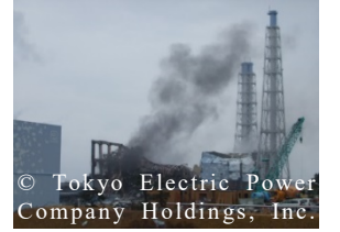
Unit 3 immediately after the hydrogen explosion
