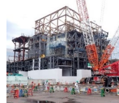
Installing a large cover for Unit 1
