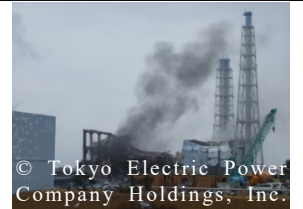
Unit 3 immediately after the hydrogen explosion
