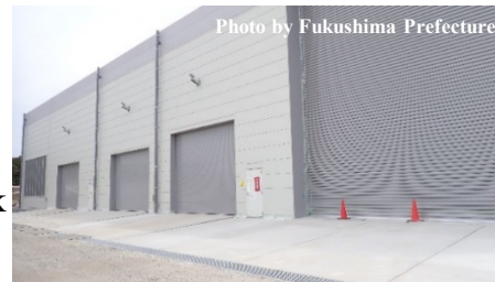
External view of the volume reduction facility
