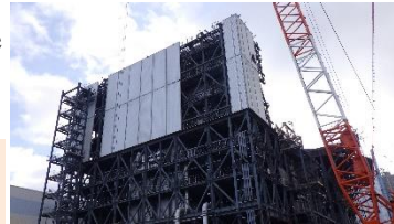
Installing a large cover for Unit 1
