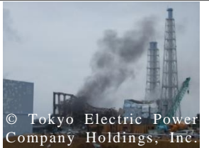
Unit 3 immediately after the hydrogen explosion
