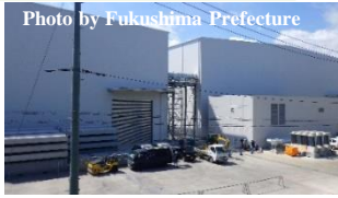
Exterior view of solid waste storage 10 (left: Building B; right: Building A)
