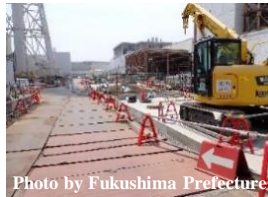
Before facing (near Unit 3)
