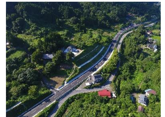
National Route 349 (Otsunagi District in Kawamata Town) In service as of 21 Mar. 2023
